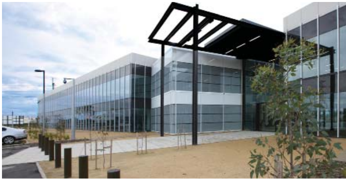
The new state-of-the-art AWD Systems Centre at Techport Australia, Osborne.
