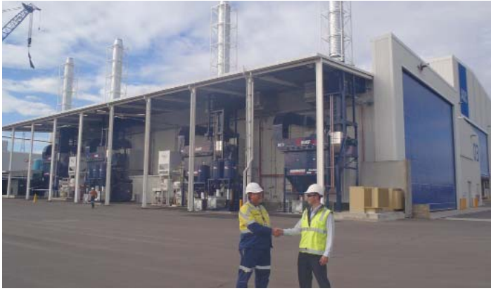
Darryl Penny, Production Senior Supervisor Blast and Paint (left), thanks Warrick March, Facility Engineering Senior Supervisor in front of the new facility.
