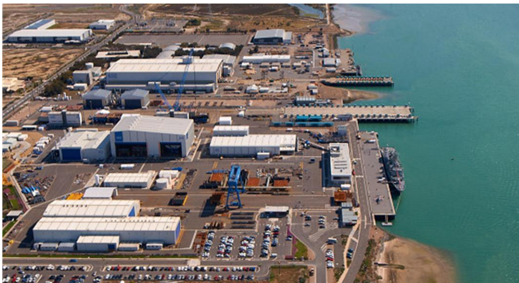
Figure 7: Modern warship and submarine integration facilities at Osborne.
